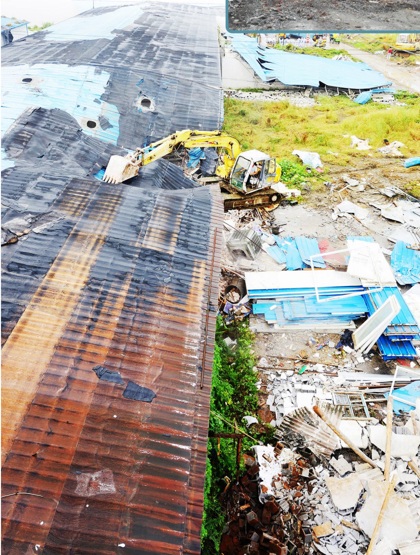
长丰决拆违现场。黄瀚 摄
